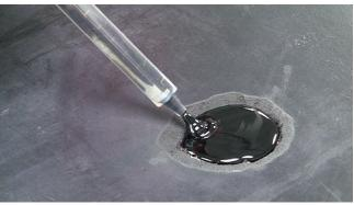
8. Dispense enough REMA GOO into the area to completely fill damaged area. Use a spreader or putty knife to smooth out material around repaired area.
