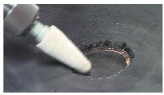
2. Grind a bevel around the gouge, hole or damaged area on the covers of the belting using a coarse grinding disc to grind 2" to 3" beyond edges of damaged area.
