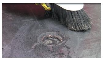
3. Use oil-free compressed air to blow off all debris or use Foxtail Dust Brush to remove debris generated during grinding. Again thoroughly clean the repair areas lightly with solvent and let the area dry completely.
