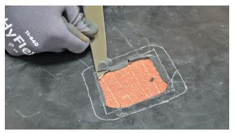
5. Bevel ½" outer marking line down to the fabric on each side using a 6" knife.
