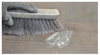
1. Remove debris and loose material from damaged and surrounding area to prepare area for buffing.
