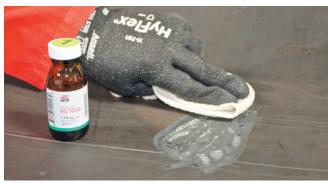
2. Liberally apply RG 7000 cleaning solvent to entire area to be repaired and extending 2" beyond area, ensuring all contaminants on belt surface are removed. Do not saturate any exposed fabric. Allow solvent to dry.
