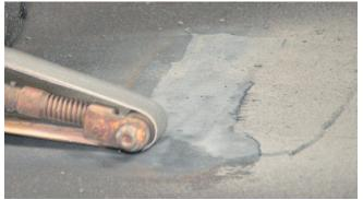
11. If desired, RG 7000 may be buffed at low speed to create a smooth surface 1 hour after application.\*
