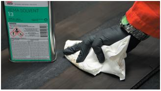
3. Liberally apply cleaning solvent to entire prepared surface, ensuring all contaminants creating during buffing are removed. Allow to air dry until it evaporates off.
