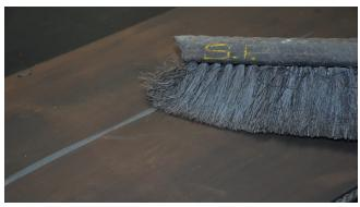
1. Using a Foxtail Dust Brush, remove debris and loose material from damaged and surrounding area to prepare area for buffing.
